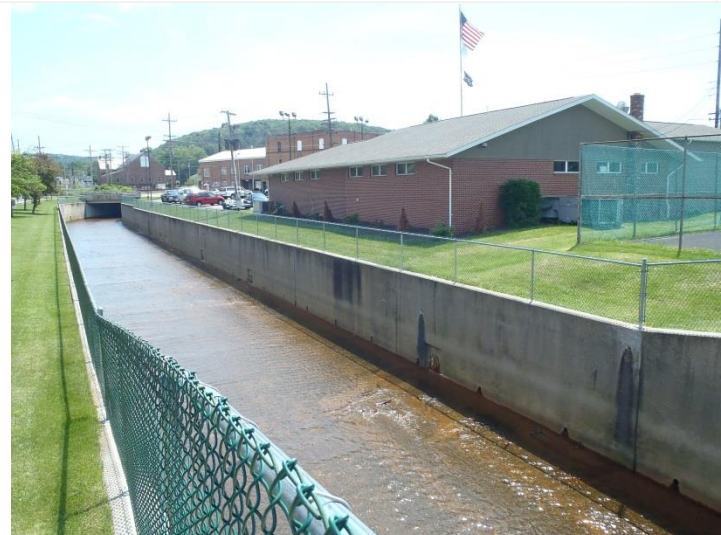
Outfalls along the Levy
