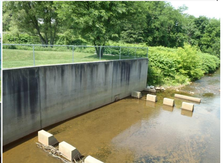
Outfall along the Levy
